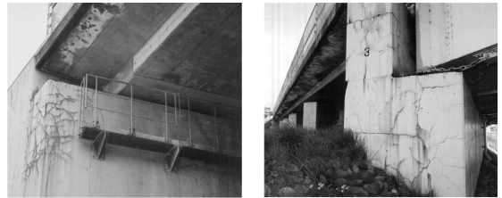
Fig.4 Alkali-aggregate reaction.
