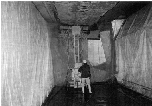
Fig.15 Removal of slab by water jet robot.
