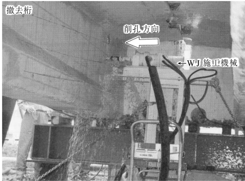
Fig.19 Drilling of PC bridge.
